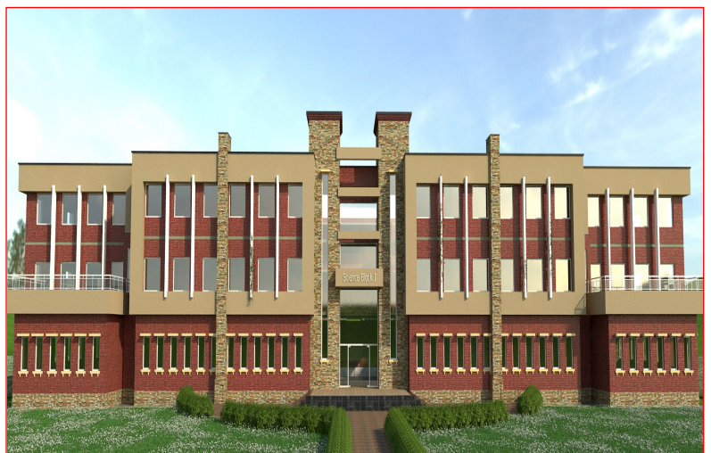
Construction Supervision of Science Block at University of Malakand Chakdara (KPK)
