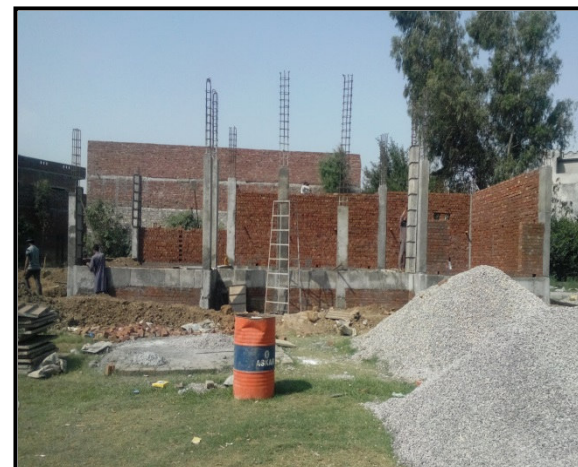
Construction of Pavilion in District Gujranwala
