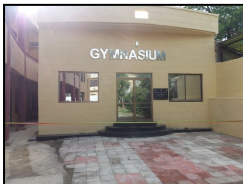
Construction of Gymnasium District Rawalpindi
