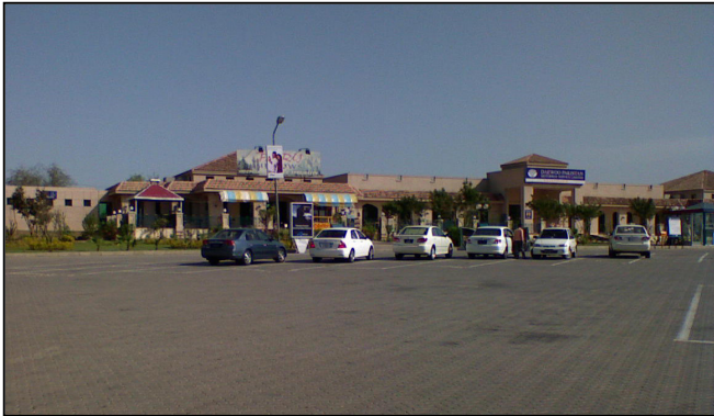
View of Chakri Service Area
