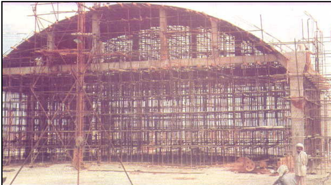
Ware House under construction
