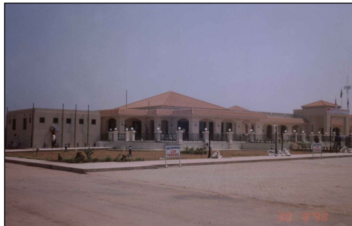
View of Bhera Service Area
