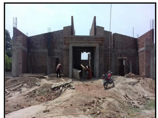
Construction of Pavilion in District Rawalpindi
