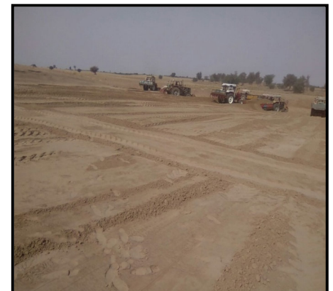
Backfilling of Cricket Ground in District Rawalpindi
