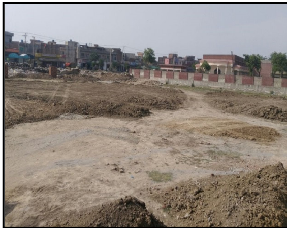
Construction of Cricket Ground in District Sarodha
